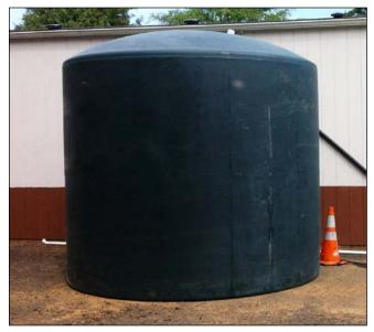
**Figure 12.** Polypropylene water storage tank with a 10,000-gallon capacity.
