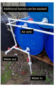
**Figure 10b.** Food-grade, 55-gallon barrels connected for rainwater storage and delivery. The filter system is separated from the storage tank, but filtered water is piped underground to the storage barrels. The collection and filter system must be higher than the storage barrels.
