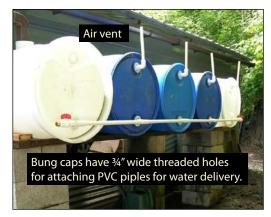
Figure 10c. Alternate way to connect food-grade, 55-gallon barrels in a series for rainwater storage and delivery. Bung caps used for securing contents of the barrels have ¾-inch pipe threads to easily connect PVC pipes for water delivery.
