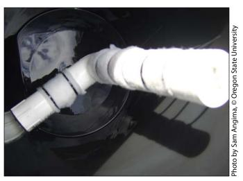
**Figure 9a.** A clean homemade rainwater-filtering system using normal household air and dust vent filter material fastened to a perforated PVC pipe.
